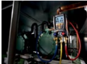
Conduct leak test
